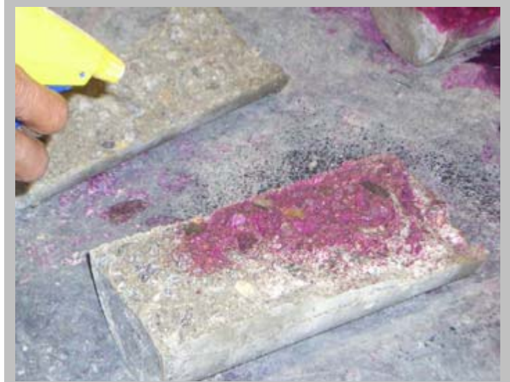
Chemically binding carbon dioxide in the concrete helps reduce emissions. Here, researchers test the depth of carbonation in a sample.
